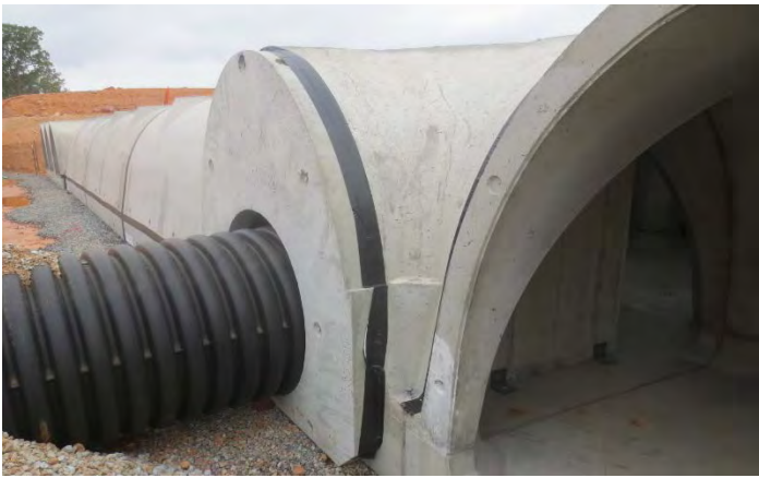
4. Install exterior piping as shown below.
