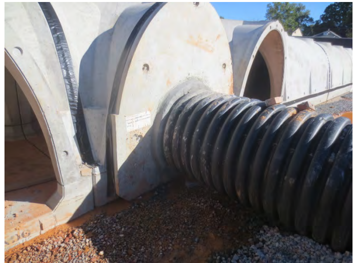
5. Grout around pipe and preformed openings on the interior and exterior surfaces as shown below.
