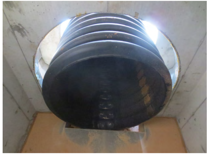
5. Grout around pipe and preformed openings on the interior and exterior surfaces as shown below.
